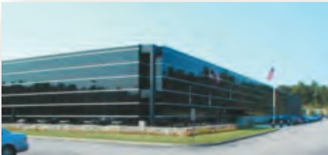
Pollak's® Canton, Massachusetts manufacturing plant.
